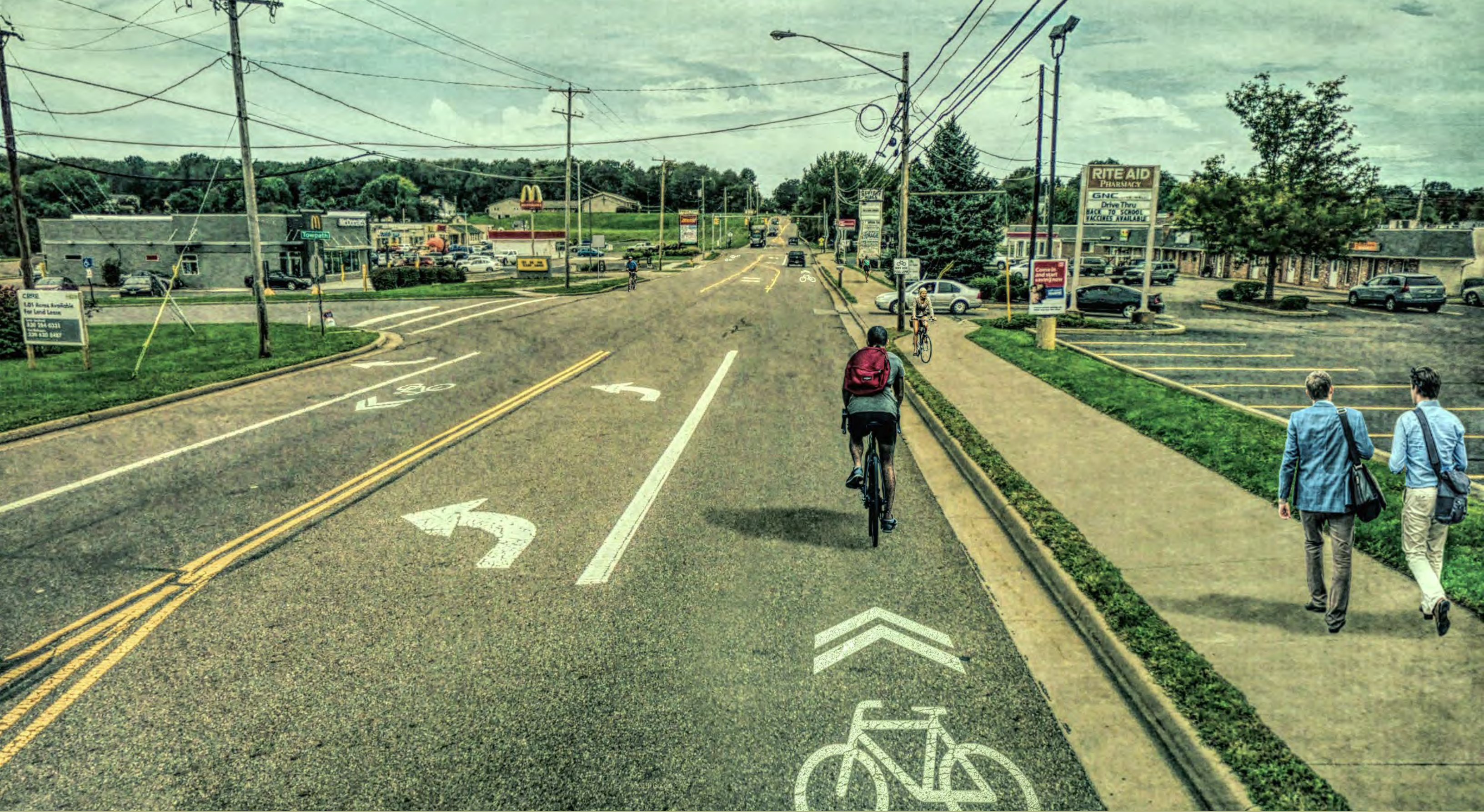
LOCUST STREET | AFTER - WIDENED SIDEWALK
